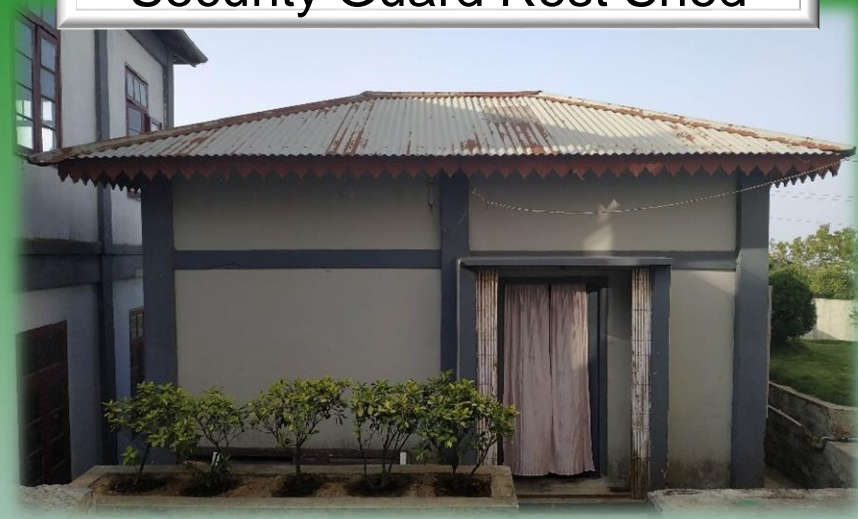
Security Guard Rest Shed
