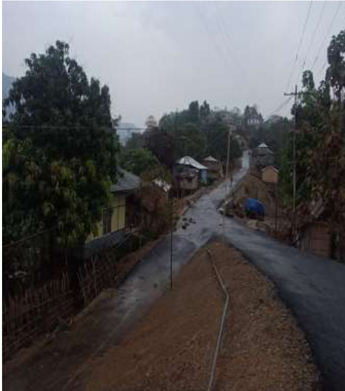
Black topping of road at Tuipuibari, Kawrtethawveng RD Block, Mamit District (Amount- Rs 140.00 lakh)
