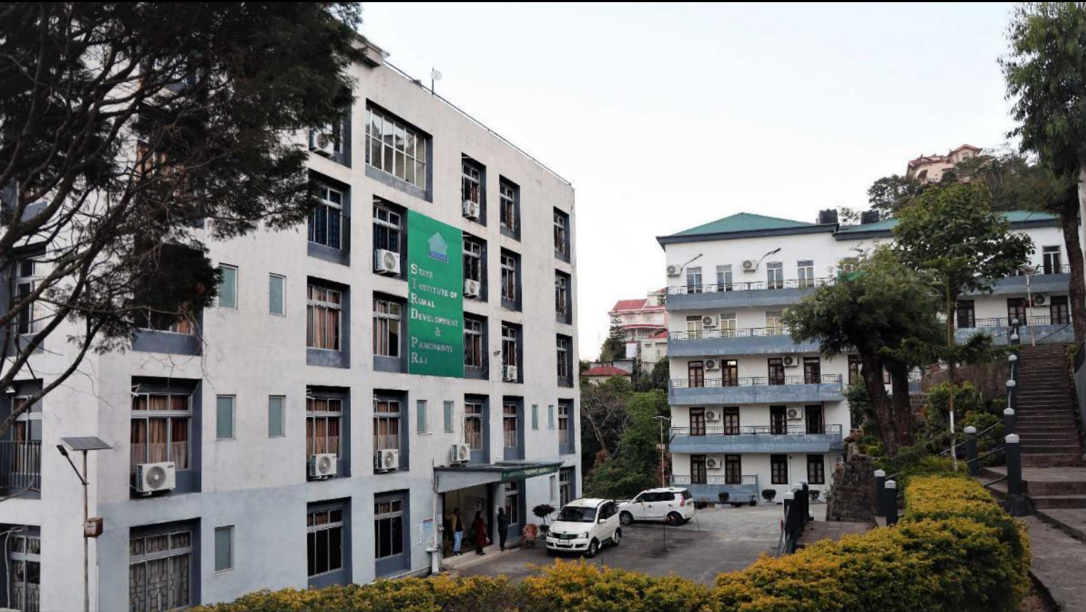
SIRD&PR Administrative Building & Hostel Durtlang Leitan, Aizawl
