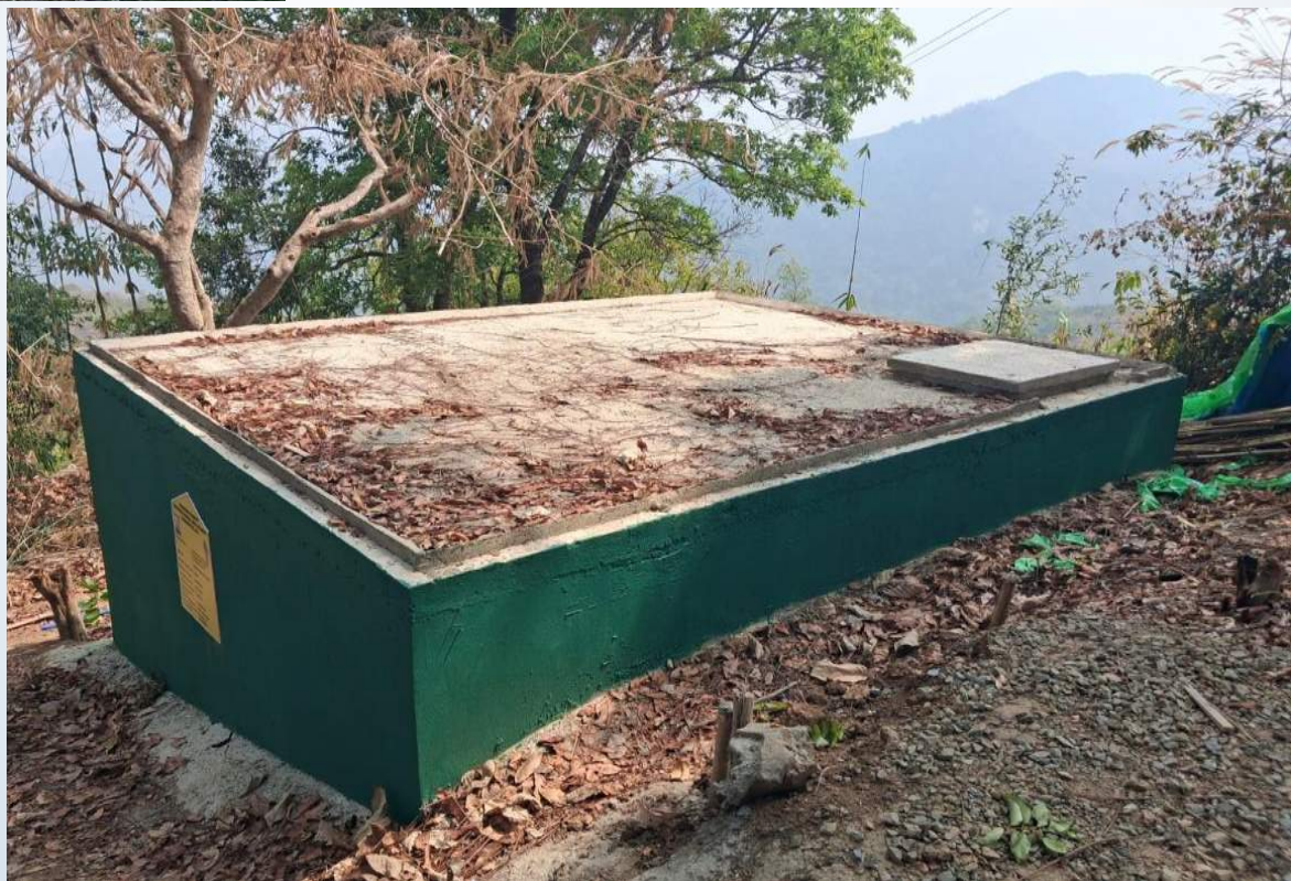
Construction of water tank at DIET Complex, Chanmari, Serchhip
